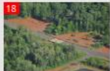
18 Hwy 2 Ashland County, WI flooding.
